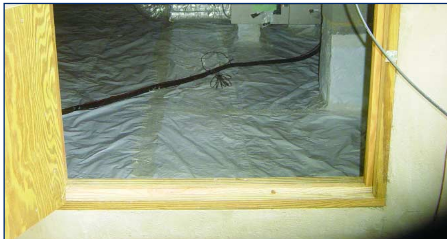
The entrance to this closed crawl space is elevated well above exterior grade, reducing the likelihood of water entry in heavy rains or minor flooding. Photo credit: Indoor Environmental Systems.
