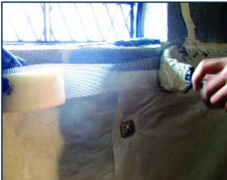
This heavy-duty vapor retarder material is mechanically supported by metal pins with cap washers and sealed to the masonry with fiberglass mesh tape and duct mastic. Photo credit: Indoor Environmental Systems.
