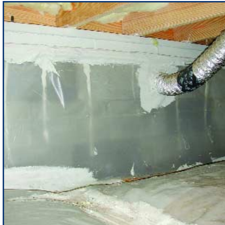
Vapor retarder material is attached with a furring strip three inches (76 mm) below the top of the masonry wall and sealed to the wall with mastic. The wall vapor retarder material is sealed to the ground vapor retarder to form a continuous liner. Penetrations, like the dryer vent in the photo, are completely air sealed. The top of the masonry wall and the front edge of the sill plate have been painted white with mastic to improve inspectability by pest management professionals.
