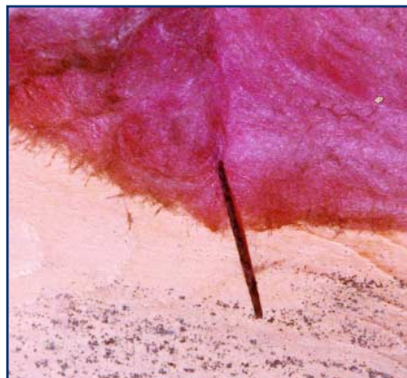
After noticing light mold growth on floor joists in a wall-vented crawl space, a contractor recommended installation of a powered crawl space ventilation fan to “dry” the crawl space.
